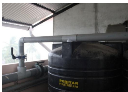
A rain water syringe for recharging groundwater, developed by Mr K J Antoji, Cochin , Kerala
