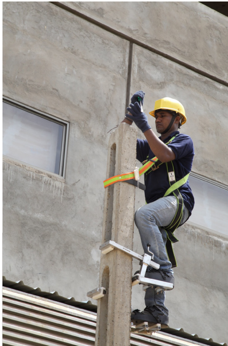
Need based Grassroots innovations for remote locations translating into strong business opportunities - The case of Pole Pro, an industrial safety device by a grassroots innovator from Kashmir valley
