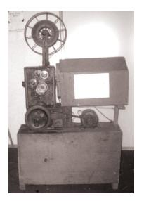
lower as it uses less power as it runs using a high powered lantern or hurricane lamp. Further the projector also has lesser number of parts and complexity than imported machines.
